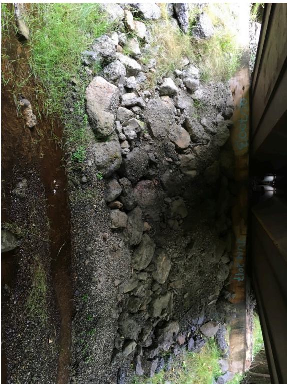
Left Bank Abutment when facing downstream
